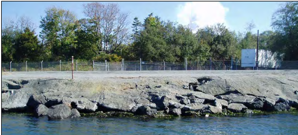
Figure 17. Lack of an upper beach and armoring immediately down-drift (southeast) of the large concrete boat ramp in cell SK-E-4. (CGS field photo)
